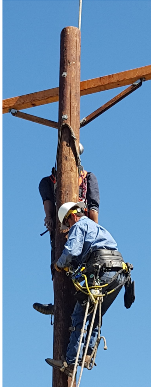
Above, Journeyman Justin Huston working a mock rescue of an unconscious line worker 25 feet in the air using only his climbing tools to make a controlled, pole top descent of the 180lb mannequin to the ground crew waiting below.
